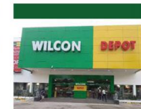
Wilcon Depot Puerto Princesa, Palawan
